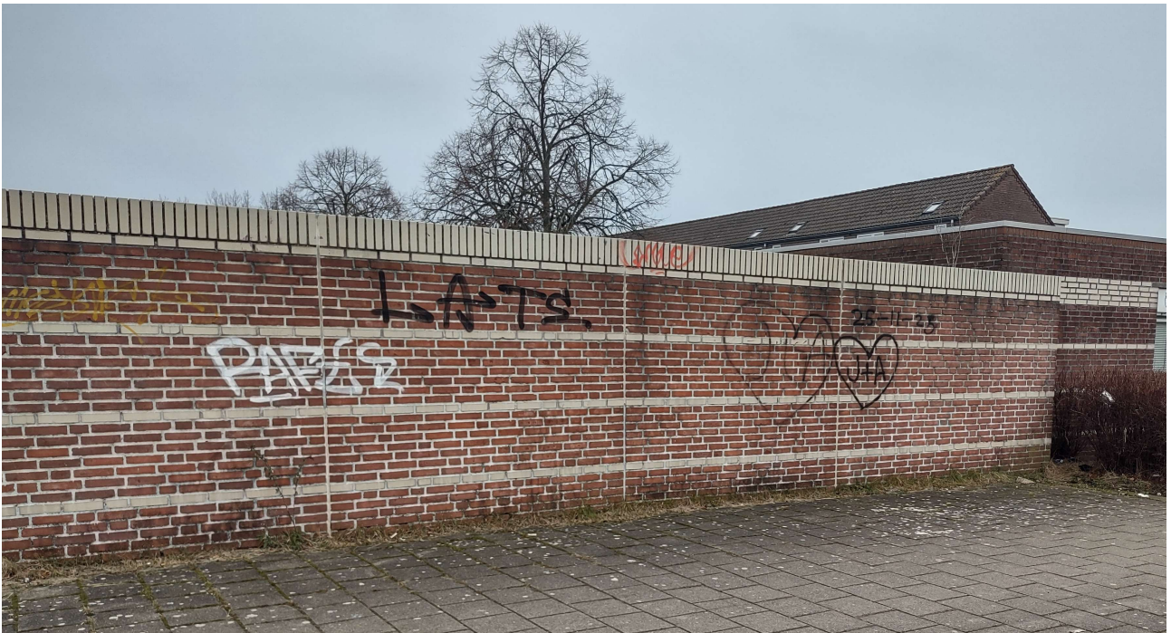
The protecting wall (to the soldiers' backs).
