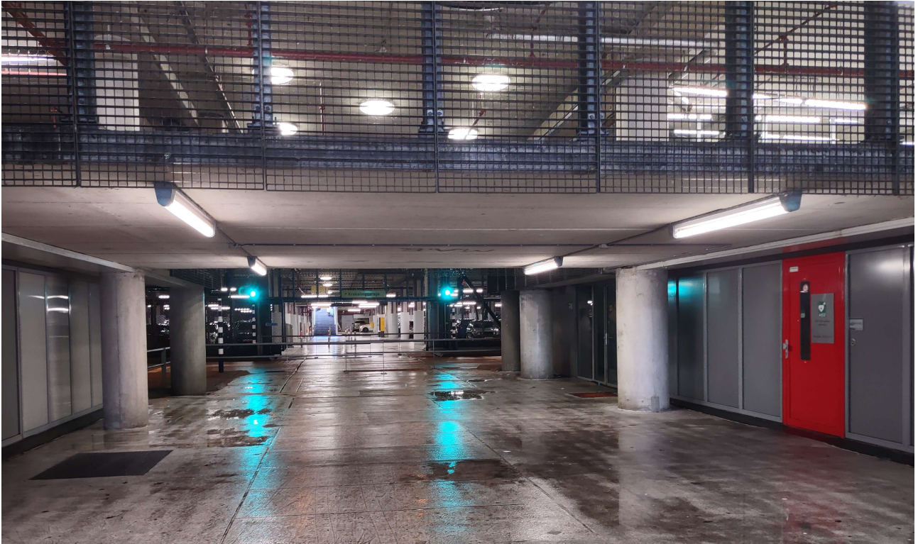
The two levels of the former casemates (now used as a parking)
