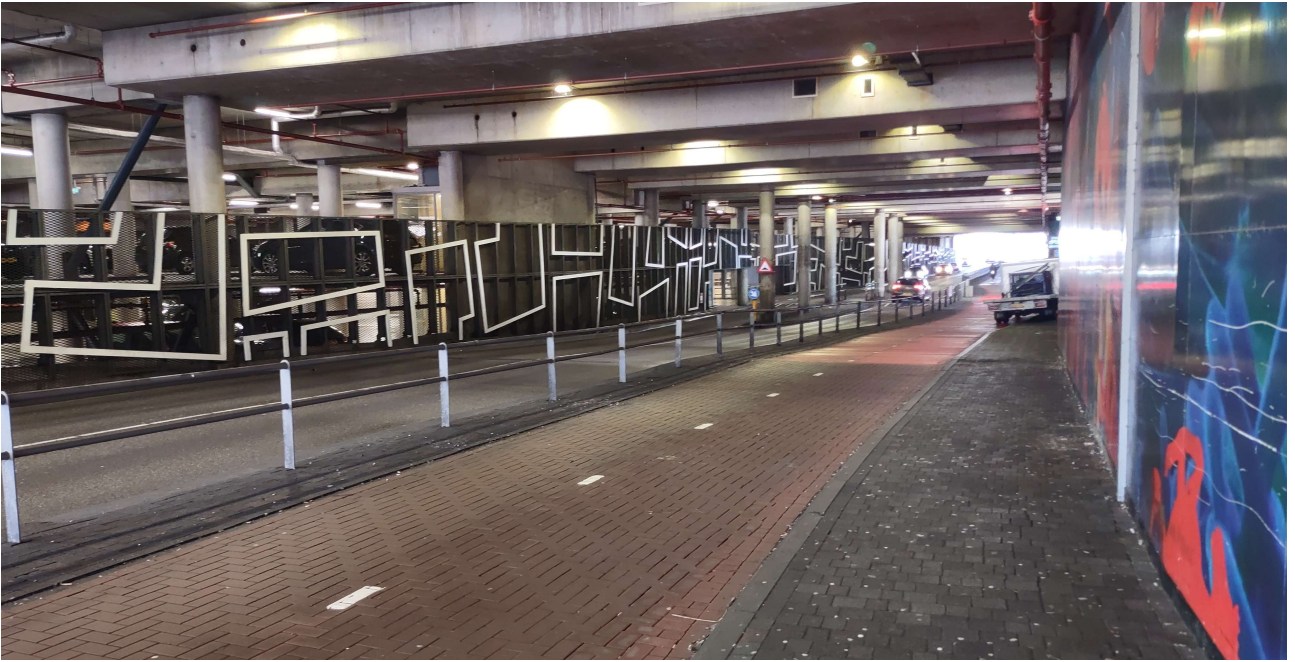
The tunnel, running through the casemates
