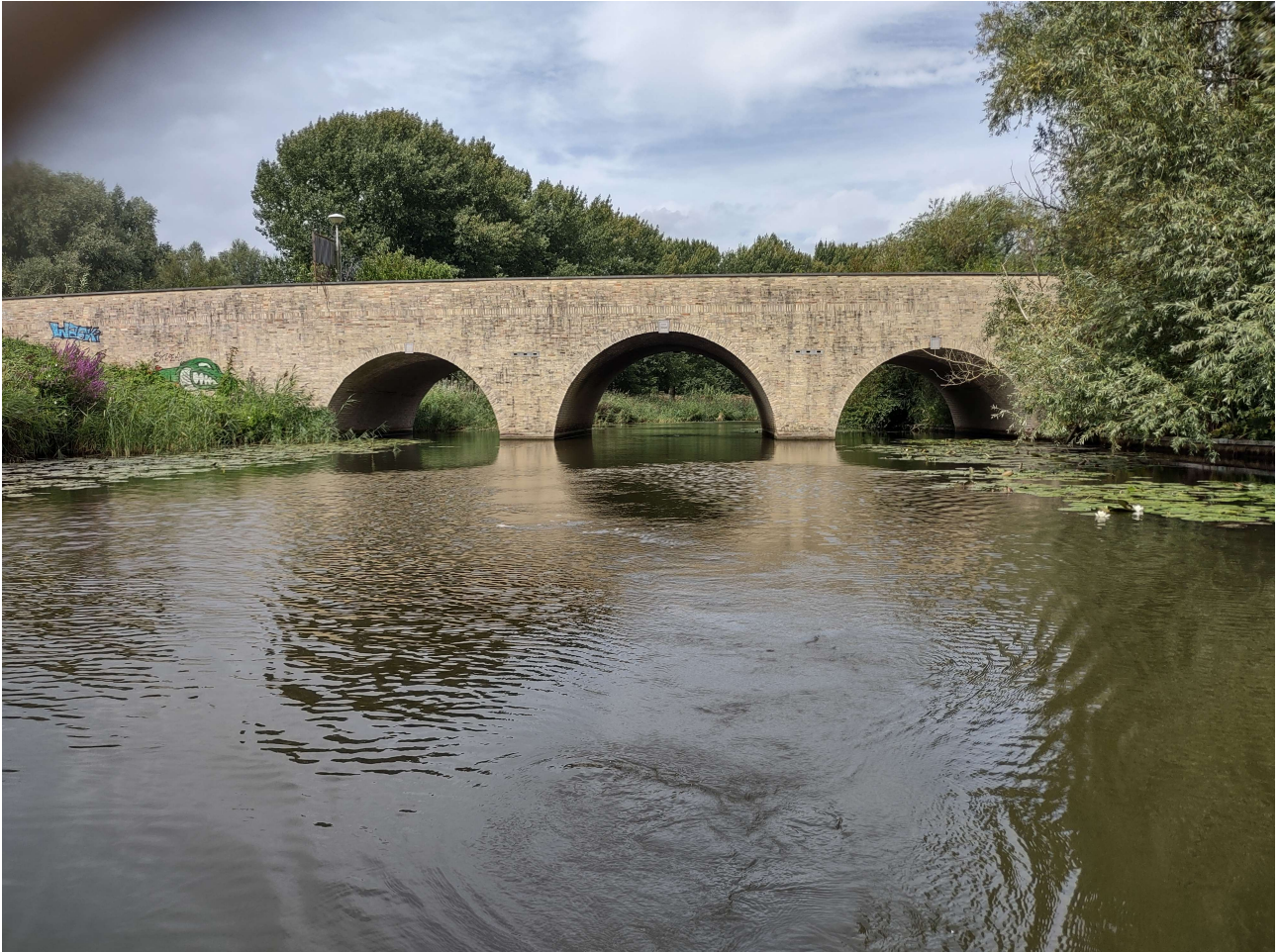
The old water gate
