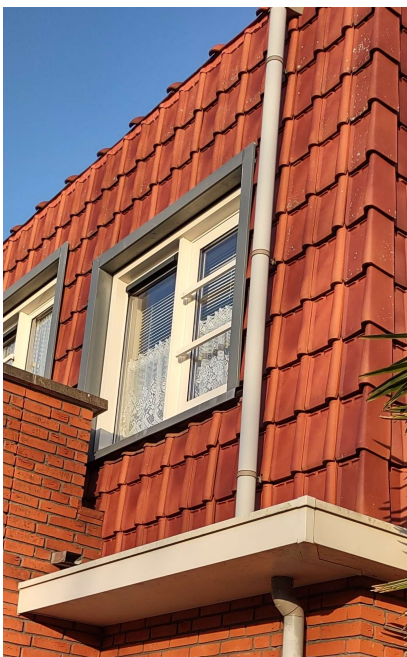
Vertical roof tiles
